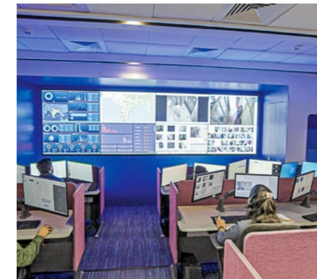
Control & Command Center, Mumbai
