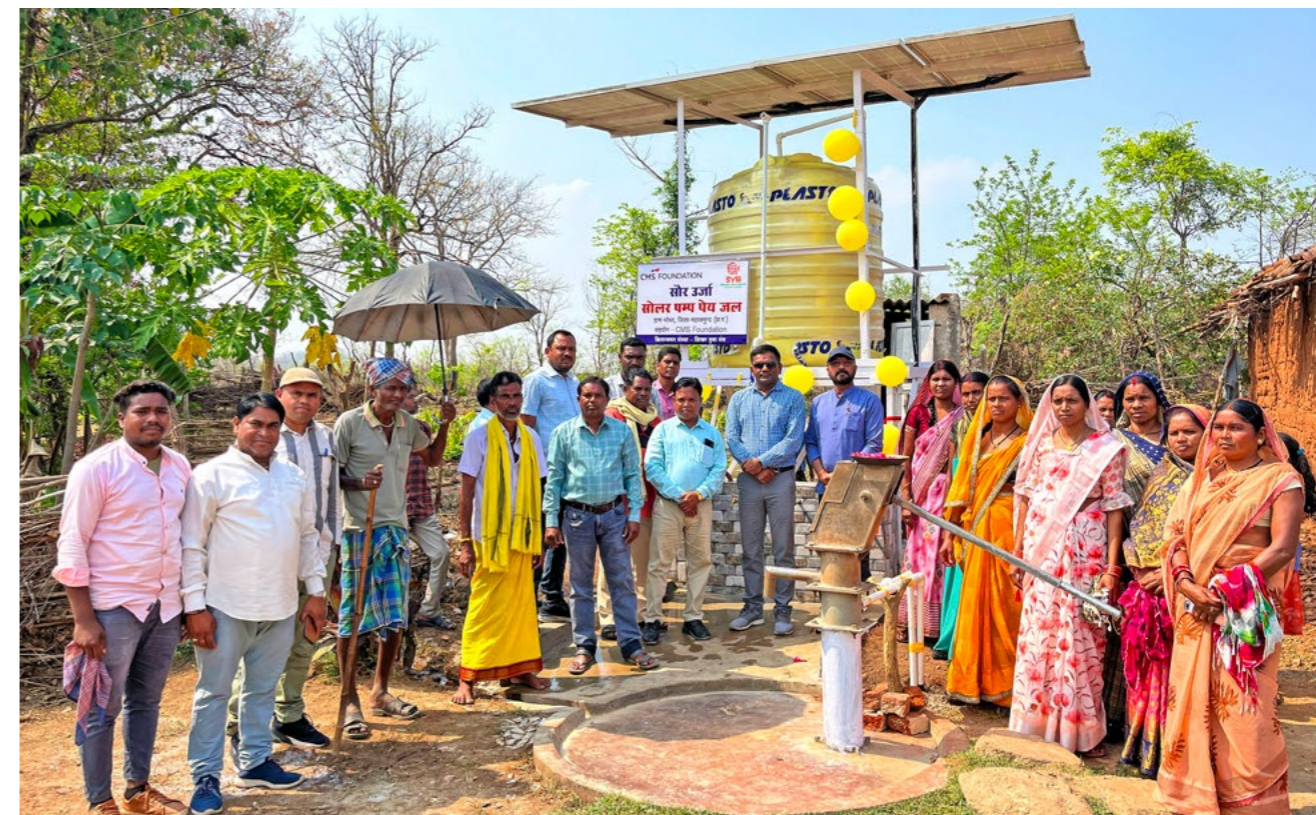
Installation of a solar-powered handpump in Bhotha Village, Mahasamundh, Chhatisgarh
